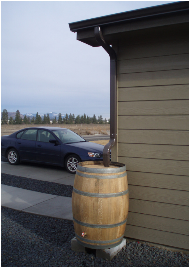
Figure 5.23 Rain barrel attached to a downspout at a Spokane, WA residence
