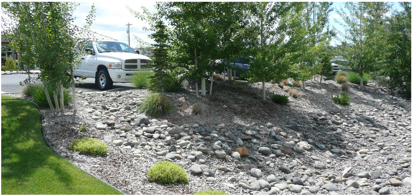
Figure 5.8 Bioretention area with rock mulch and minimal vegetation Photo by Bill Rice
