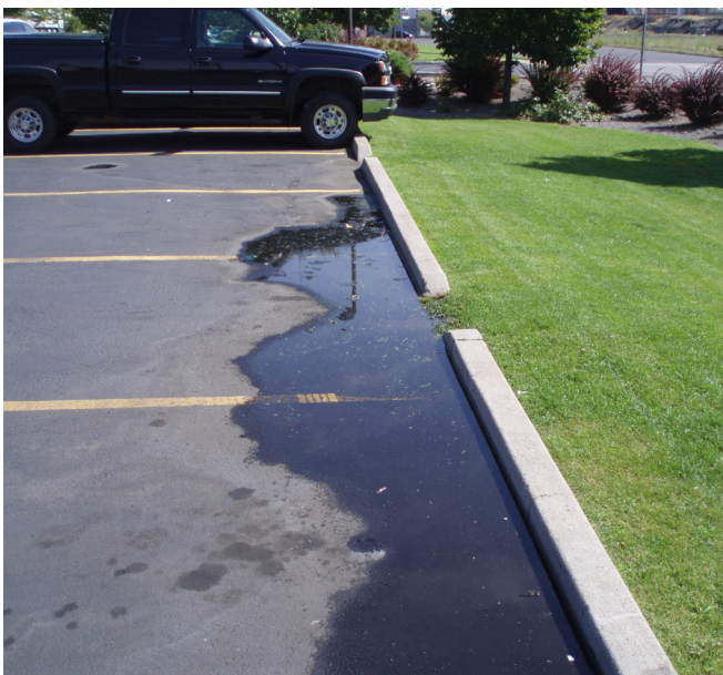
Figure 1.7 A blocked inlet on a parking lot results in pollutant accumulation and reduced groundwater recharge
