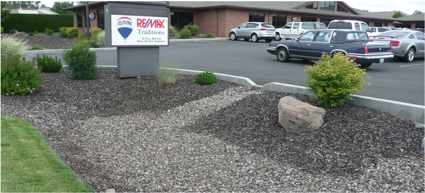
Figure 5.2 A low-maintenance bioretention area with minimal vegetation and curb cuts in parking lot Photo by Bill Rice
