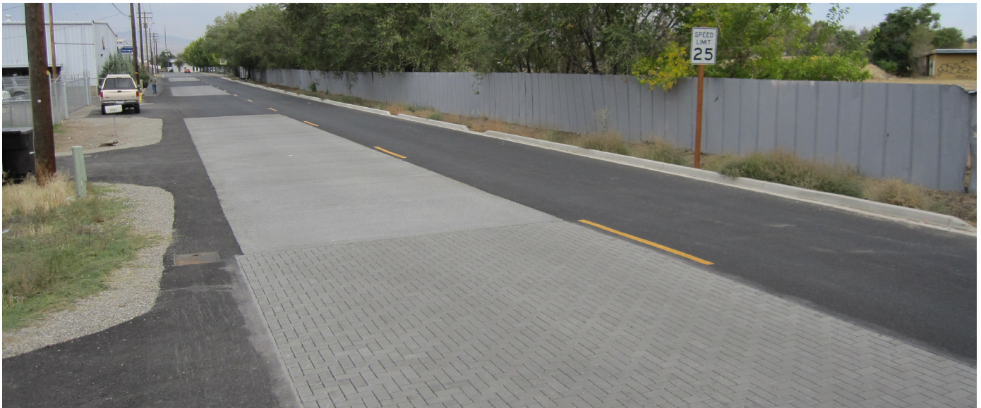
Figure 5.13 Permeable Pavers Installed at the Yakima County LID Demonstration Project on J Street, Yakima, WA Photo by Erik Pruneda
