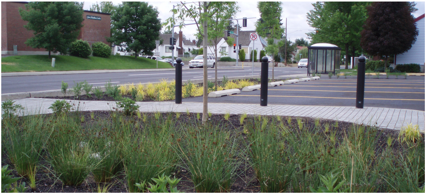
Figure 5.1 Bioretention Areas in a Parking Lot in Spokane, WA. Photo by: AHBL, Inc.
