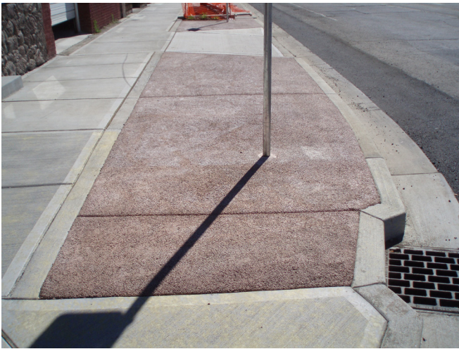
Figure 5.16 A colored application of pervious concrete
