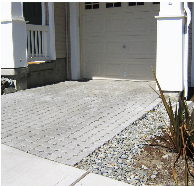
Figure 3.15 Short driveway with permeable pavers at High Point, Seattle, WA
