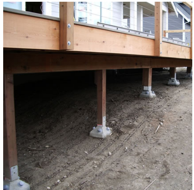
Figure 5.19 Deck and grade beam supported by pin foundations on a sloped site Courtesy of Diamond Pier®
