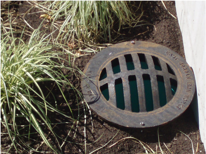
Figure 5.7 A surface drain installed at the designed maximum ponding elevation is one option for providing surface overflow
