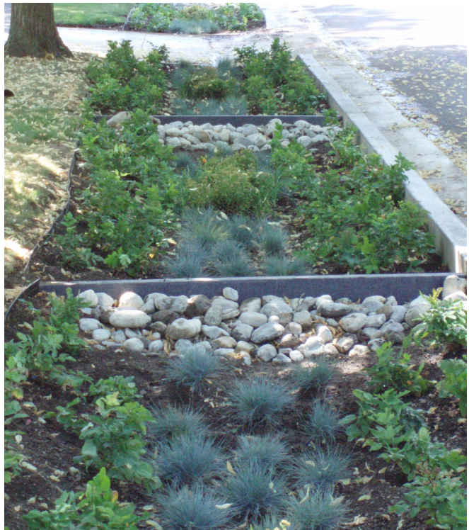
Figure 5.9 Check dams installed in a bioretention facility on a sloped site adjacent to a roadway
