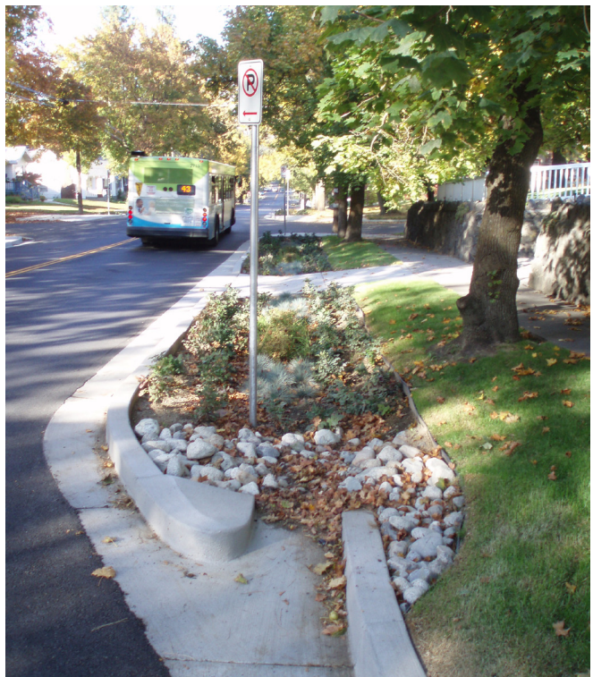
Figure 3.2 On-street parking spaces are removed to accommodate bioretention cells, Spokane, WA
