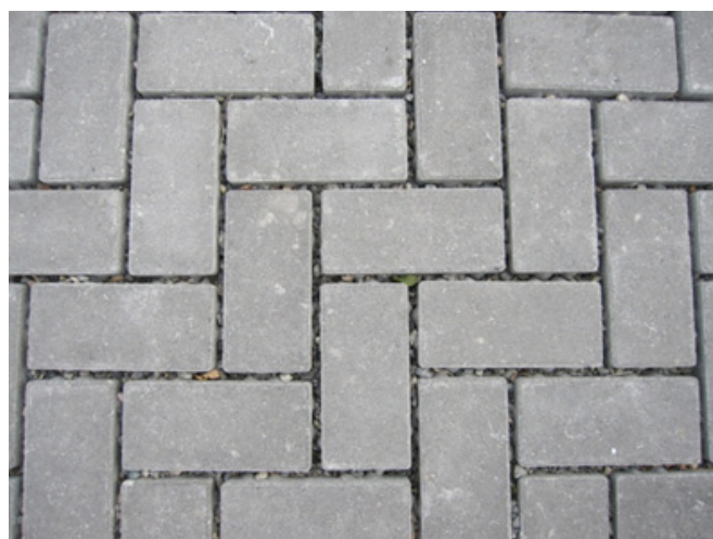
Figure 5.18 Close-up of concrete pervious pavers installed as part of the Yakima County LID Demonstration Project. Photo by Erik Pruneda
