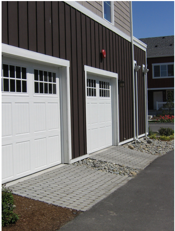
Figure 3.13 Permeable pavers used in an alley at High Point, Seattle, WA
