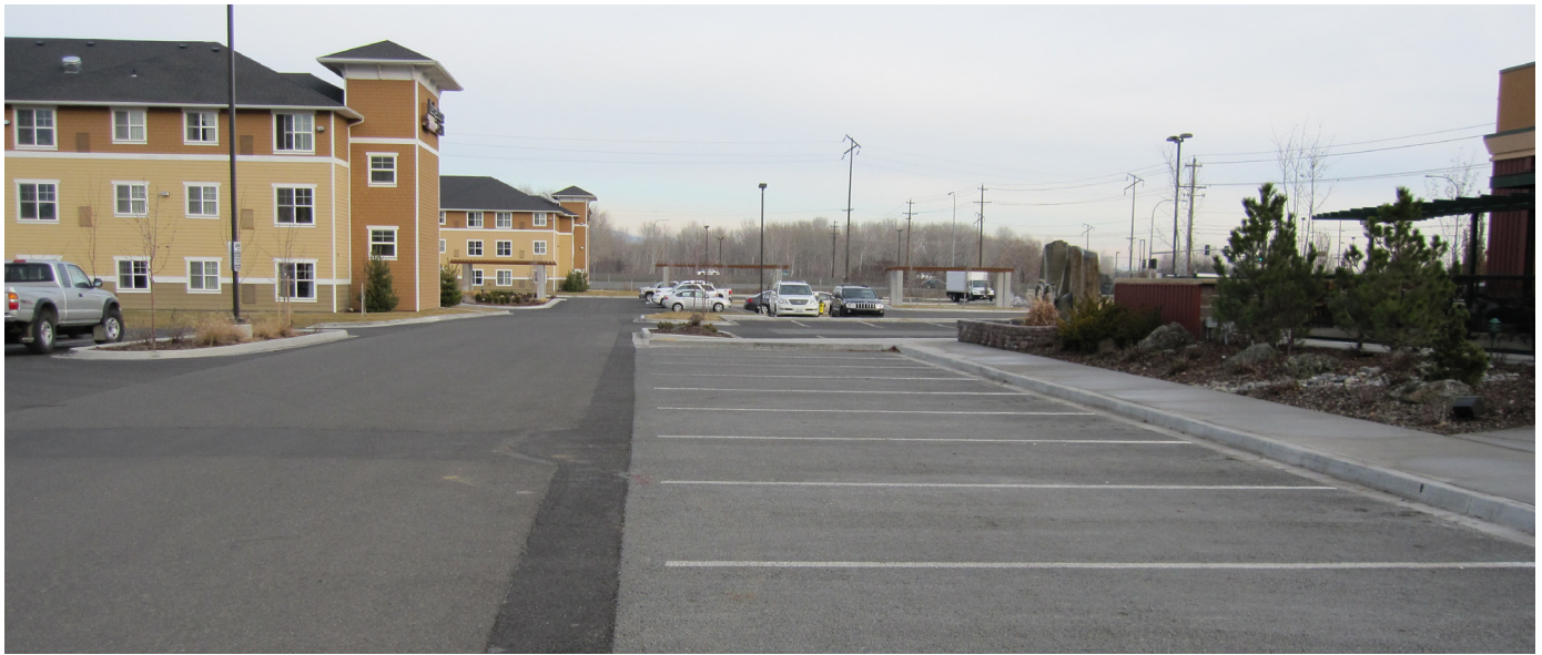
Figure 5.17 Pervious concrete installed in a parking lot application. Photo by Erik Pruneda
