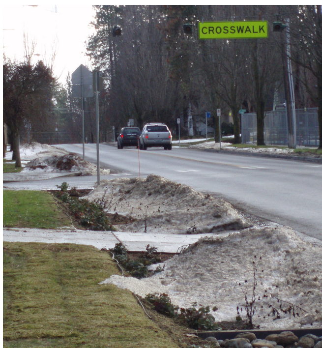
Figure 3.3 Snow storage in bioretention cells, Spokane, WA.
