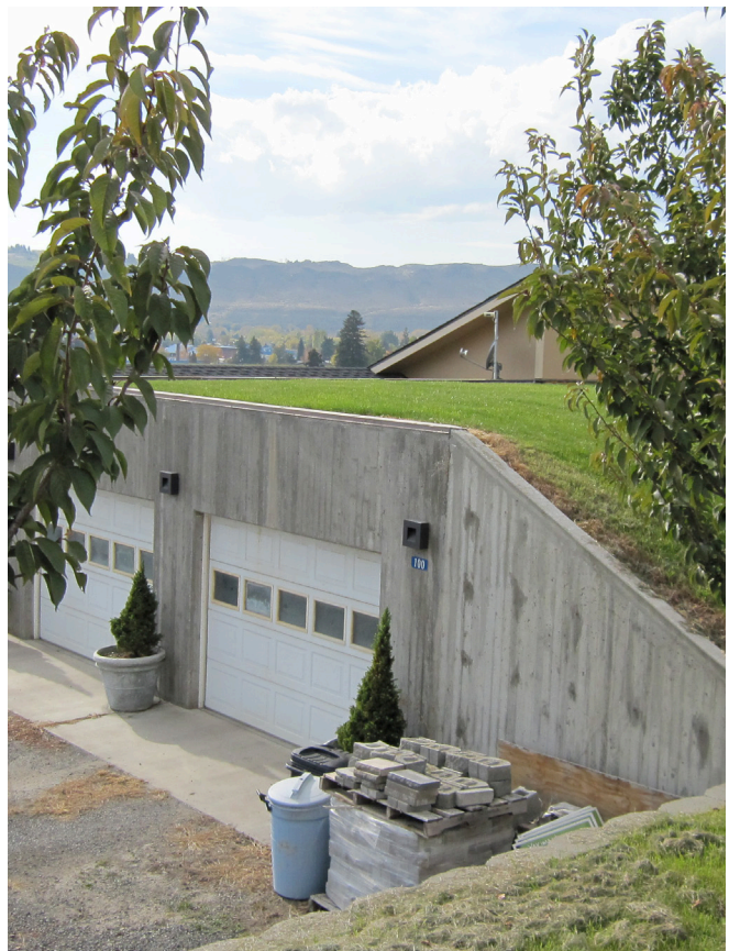
Figure 3.17 Green roof in Naches, WA. Ideally, green roof vegetation in an arid climate would be tolerant of extreme heat, shallow soils, and wind Photo by John Knutson
