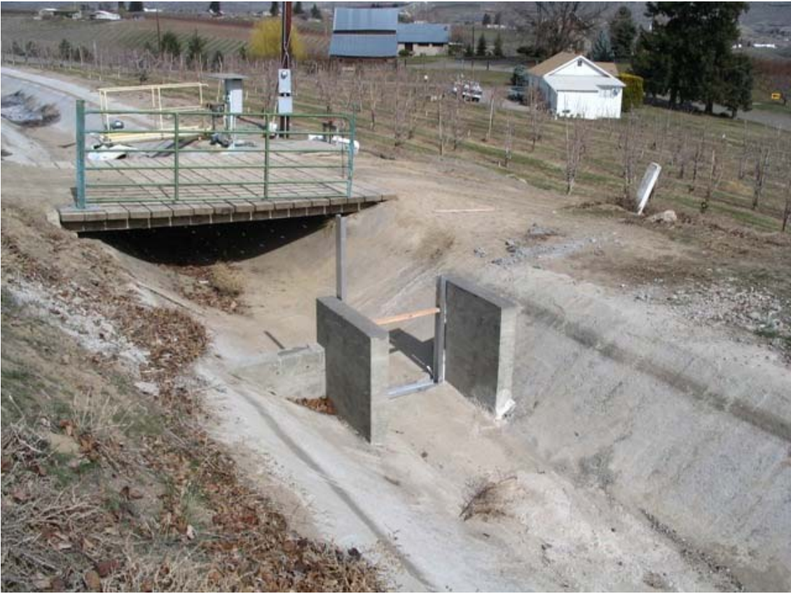
No. 2 Gate Check Structure – looking from downstream
