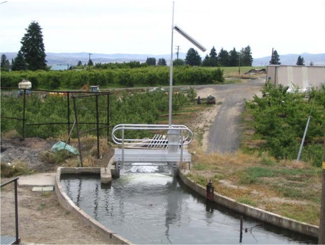
No. 1 Gate, start of the No. 1 Lateral – looking from upstream
