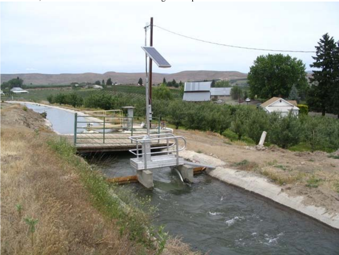
No. 2 Gate – looking from downstream
