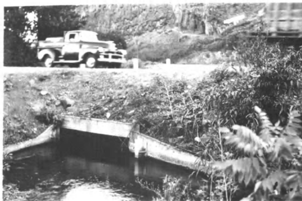
Photo No. 1. - Stop plank guides in Hubbard Canal at U. S. Highway No. 410 crossing.
