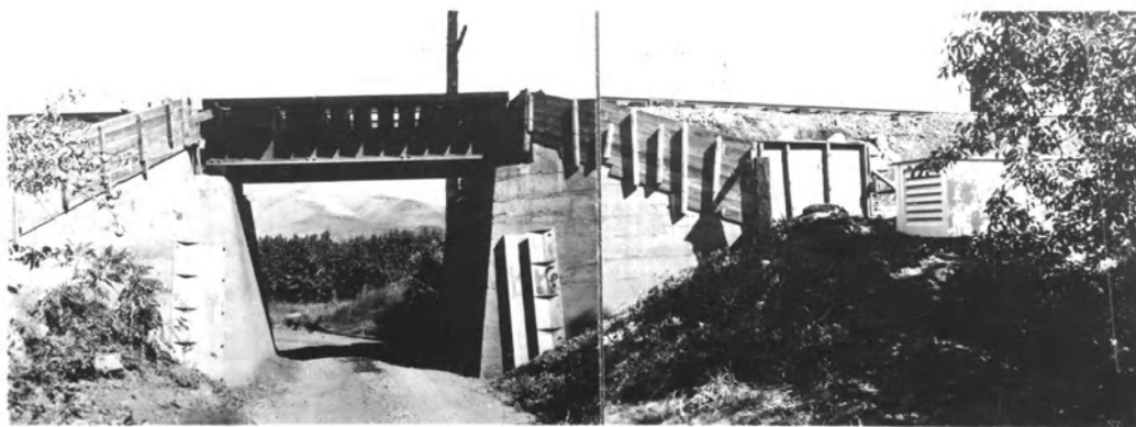
Photo No. 3. - Stop plank guides in the Northern Pacific Railway (Main Line) underpass. Note the stop log storage structure on the right side of the photograph.
