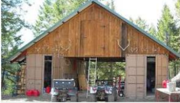
*2 cargo containers supporting a roof structure.
