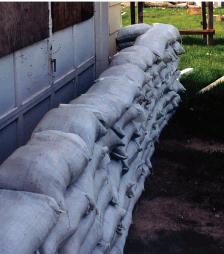
Single stack placement
