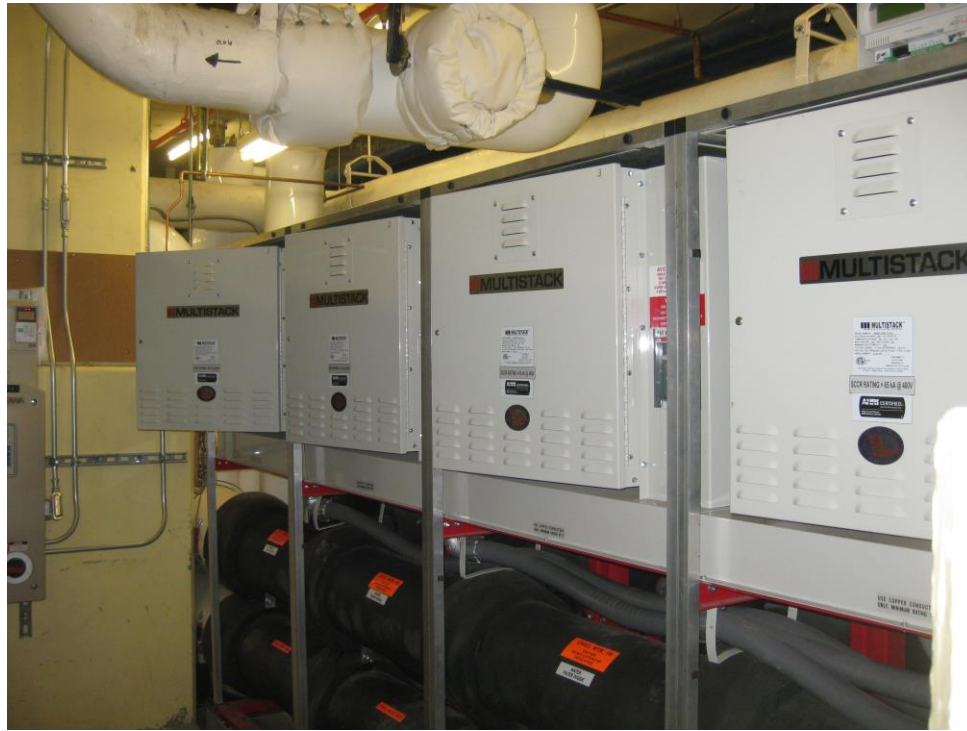
Figure 6 - Multistack Chiller
