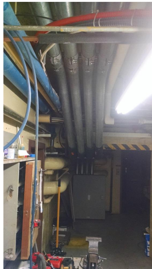
Photo 1: Power Feeders Routed Through "Old Jail"
