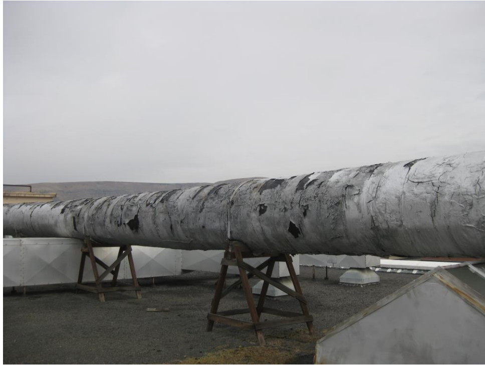
Figure 4 - Rooftop Return Duct (1941 Building)
