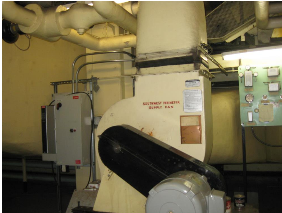
Figure 2 - Perimeter Supply Fan
