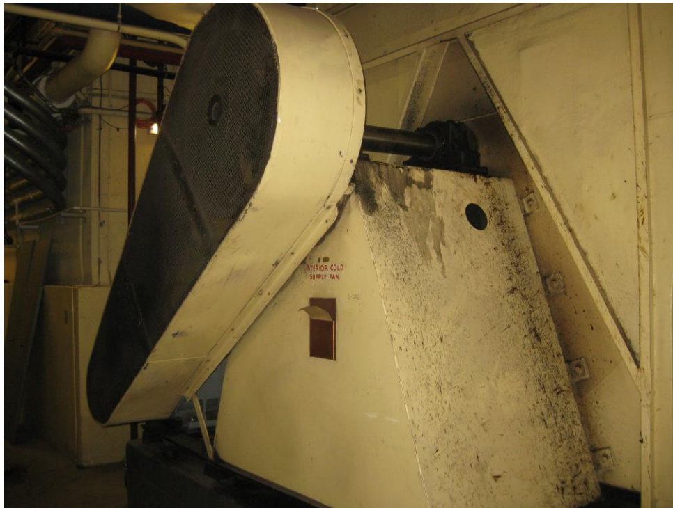
Figure 1 - Interior Cold Deck Supply Fan
