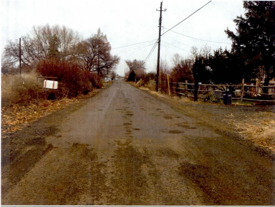
66th Avenue looking north of Annexation Area – Gravel Roadway, no curb, gutter or sidewalk
