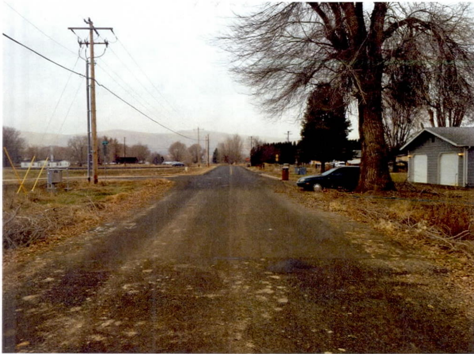
66 th Avenue looking south towards Ahtanum – Bituminous surface transitions to asphalt pavement. No curb, gutter or sidewalk north of Woolsey Road. Curb and gutter but no sidewalk south of Woolsey Road.
