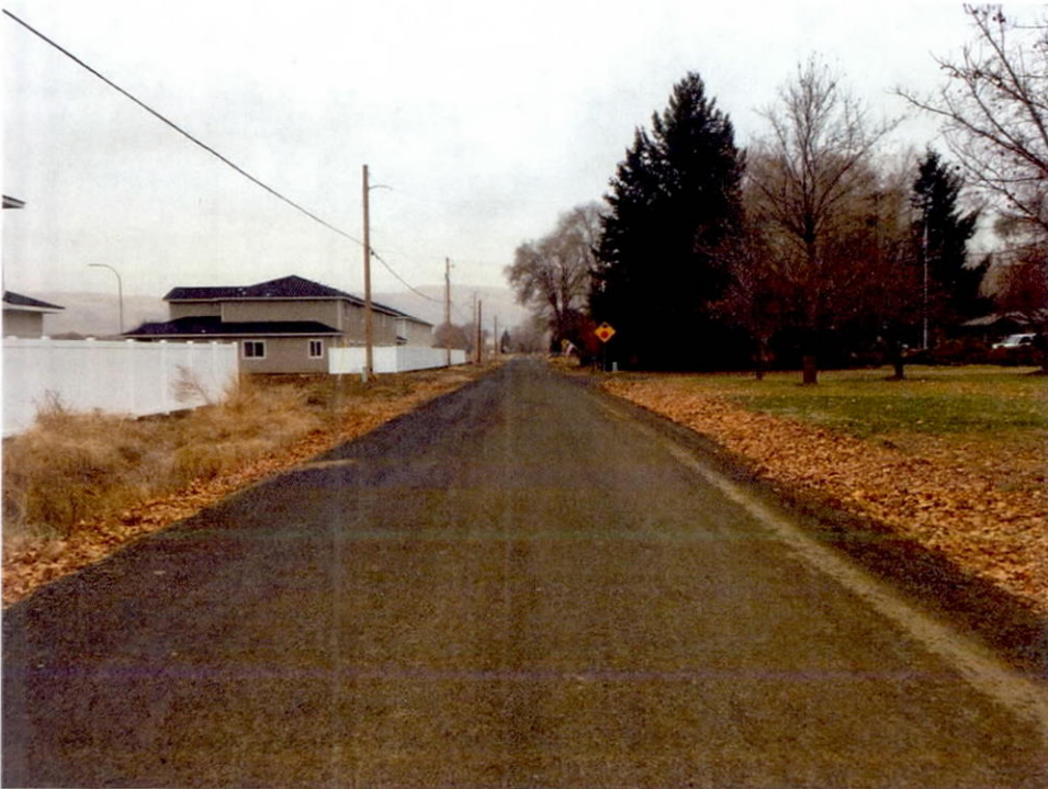
66 th Avenue looking south towards Ahtanum – Bituminous surface, no curb, gutter or sidewalk
