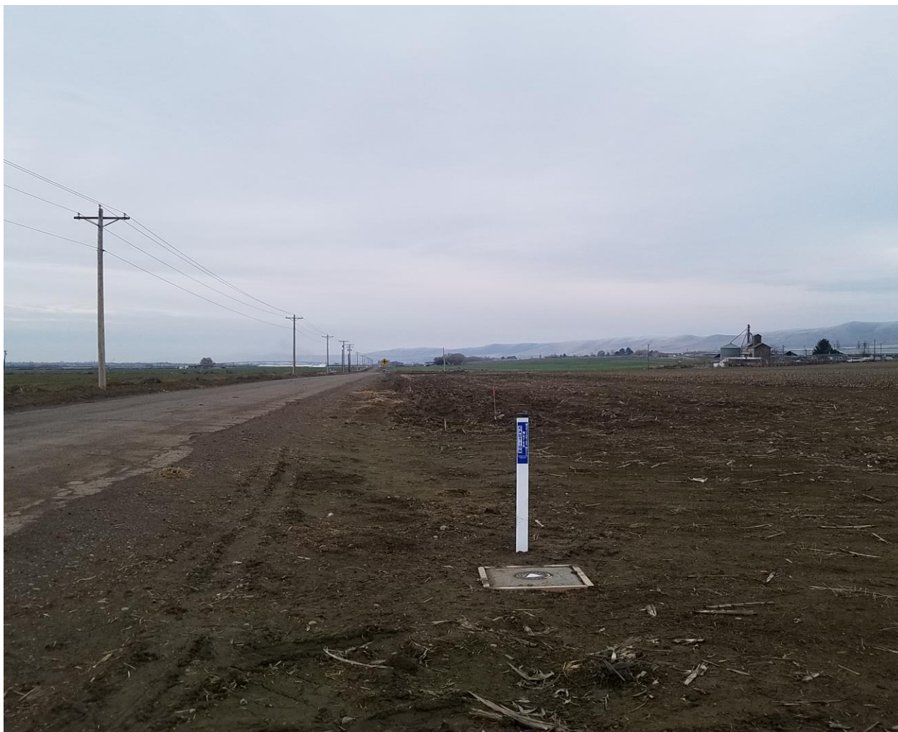
YC-MW-28 Wellhead Completion Photo
