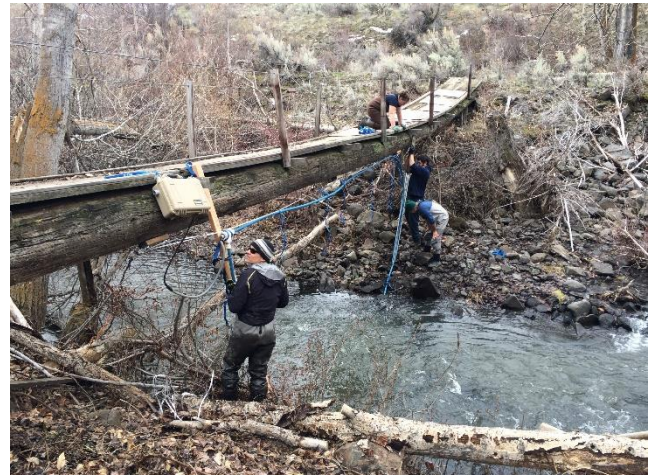
Crews install PIT antennas on Wenas Creek. Source: NYCD.
