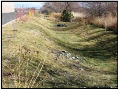
Instead of a pipe system to the nearest creek, stormwater is infiltrated onsite to mimic pre-development conditions.
