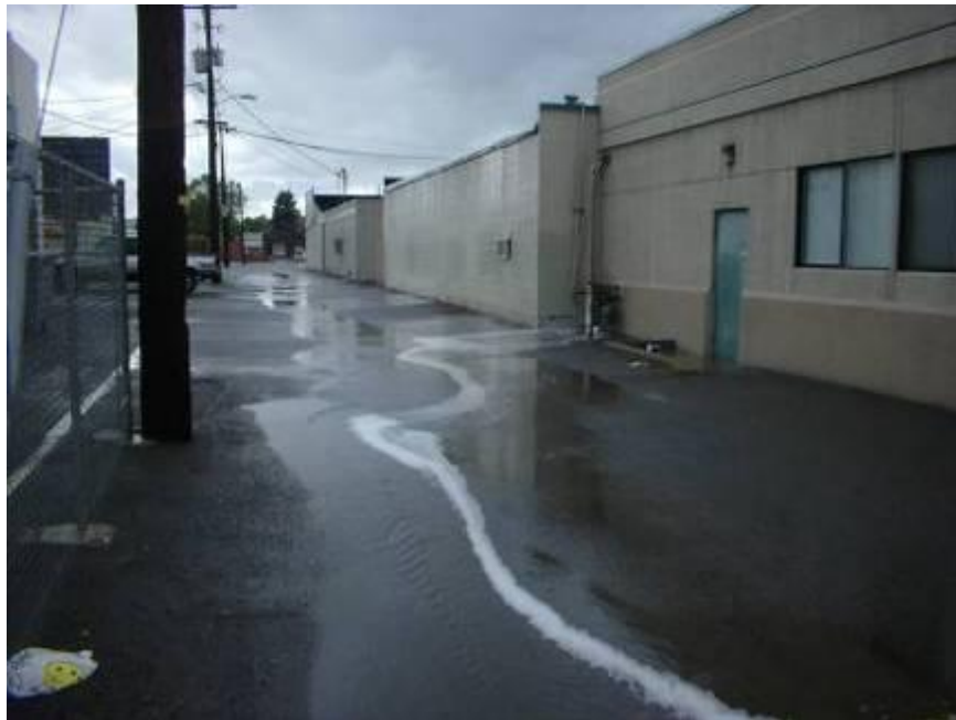
Figure 1. Stormwater runoff from a building roof.
