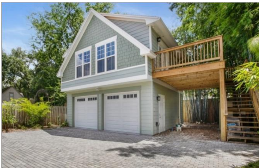
Figure 16: Elevated Accessory Residential Structure, with Enclosure
