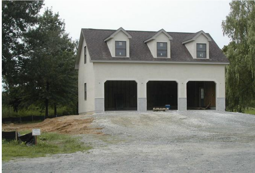
Figure 21: Three-Car Garage Elevated on Fill
