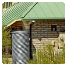
Active rainwater harvesting in Tucson, AZ.
