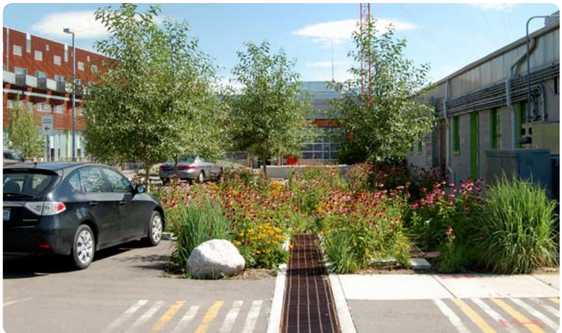
Rain gardens fed by passive rainwater harvesting border the buildings and parking lots of the TAXI redevelopment project in Denver, CO. The rain gardens beautify the site, reduce the urban heat island effect, and provide habitat, while reducing runoff to the nearby South Platte River. Photo courtesy of Wenk Associates.
