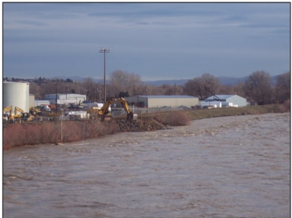
Rip-Rap Repair at NC Machinery Levee January 2009
