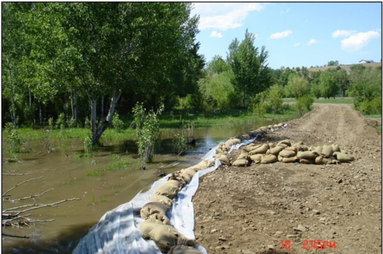
Sandbags used along Ahtanum Creek during the 2006 flood to prevent channel avulsion.
