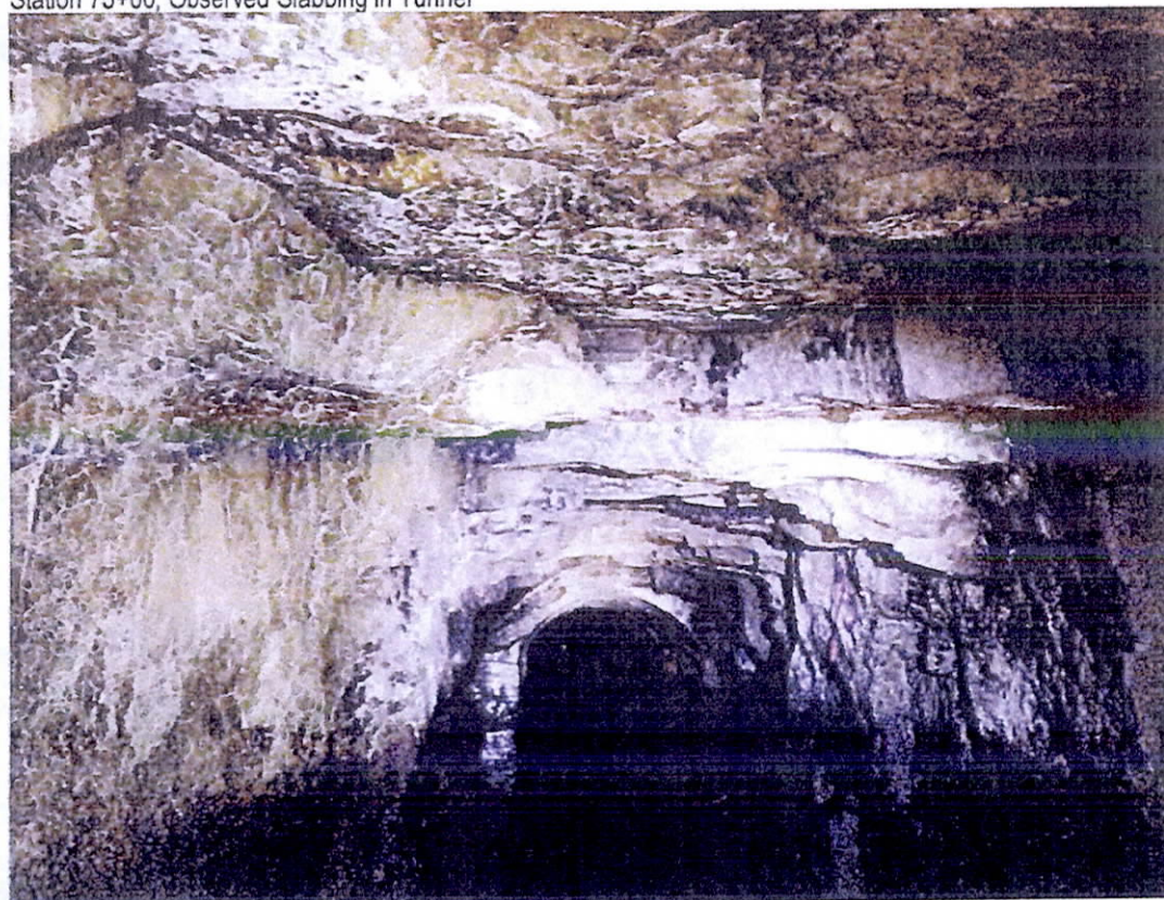
FIGURE 6 Station 75+00, Observed Slabbing in Tunnel
