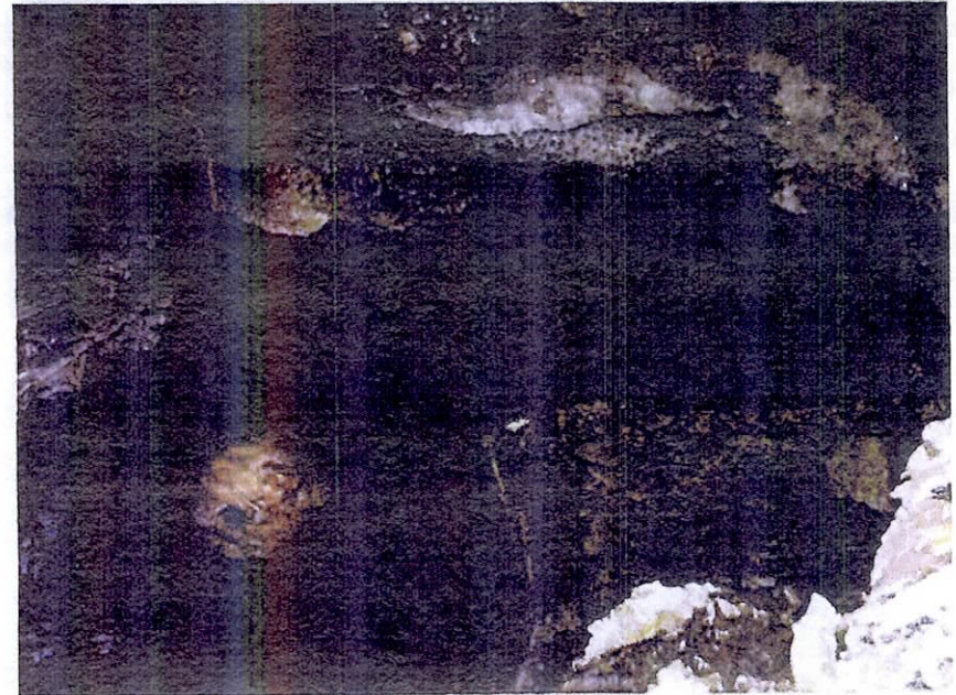
Station 74+73, Void Above Tunnel Liner
