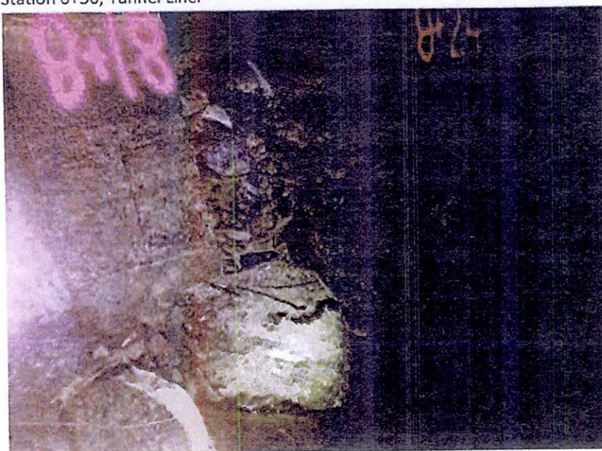
Station 8+18, Rock Block in Invert
