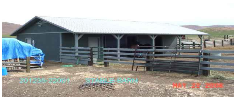
Average to Good (depending on interior amenities) .... framed construction- extra entry doors-some electrical. Use lean-to rate for open wings on each side. Good quality would include adequate lights and outlets, water service, stalls and feed room.
