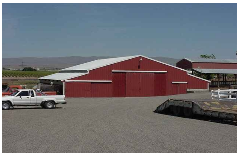
Average to Good (depending on interior amenities) .... framed construction- extra entry doors-some electrical. Use lean-to rate for open wings on each side. Good quality would include adequate lights and outlets, water service, stalls and feed room.
