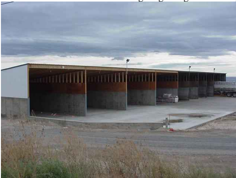
Good...tall stub walls – framed - lighting – large concrete apron.
