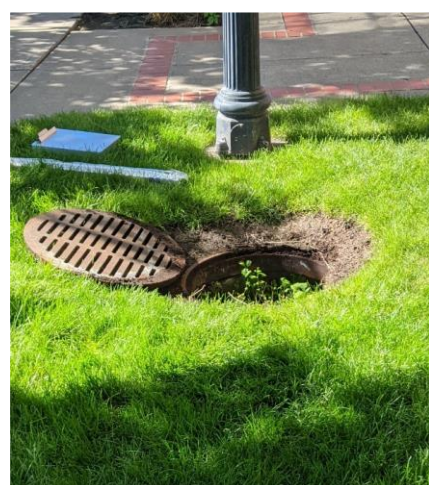
Figure 2-2. Plant growing inside drywell
