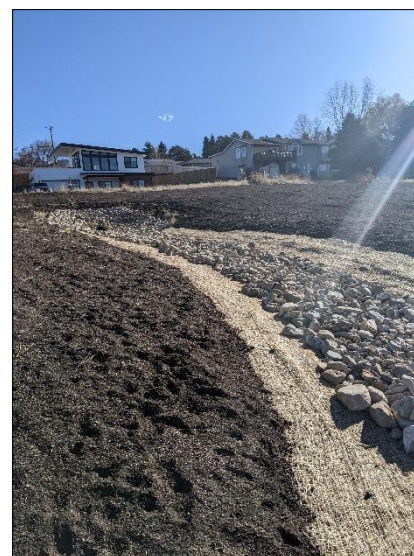
Figure 5-3. Swale leading to detention basin managed by HOA in Missoula, MT
