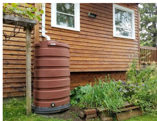
Figure 7-1. Rain garden on residential property (top) – RainWise Cistern (bottom) (source: https://www.monsoonraingardens.com/ )
