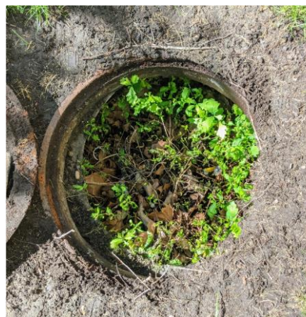
Figure 2-3. Sediment buildup
