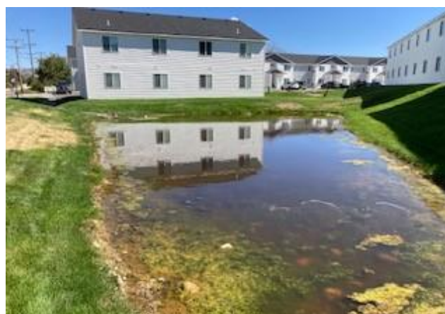
Figure 5-2. Unmaintained stormwater pond on multi-family parcel
