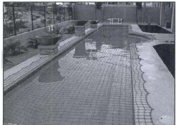
FIGURE 305.1(4) NONPOWERED MESH COVER DOES NOT ALLOW FOR ABSENCE OF BARRIER AROUND POOL
