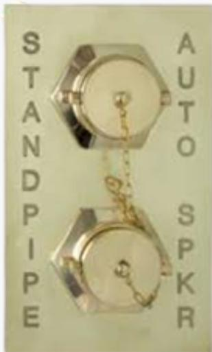
FDCs come in a variety of types and configurations. They are required to be visible from the street or fire access roadway.
