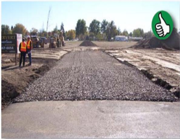
*An excellent example of a properly installed construction entrance.
