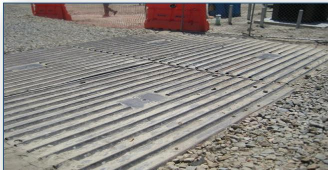
Photo: Grizzly incorporated into the Trackout Pad BMP.
