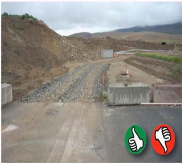
*Good installation of a construction entrance, but sediment is still being tracked off-site. Add more rock or make entrance longer.
